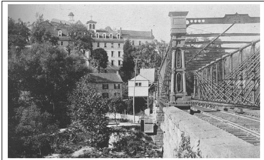
The Howard County end of the Bollman truss bridge appeared on the left edge. This iron bridge was damaged in the 1868 flood ( Gazette , July 27, 1868). The 1904 relocation of the railroad passed to the right of the mill and followed the south bank of the river. The mill ruin could not be found in January 2006.
